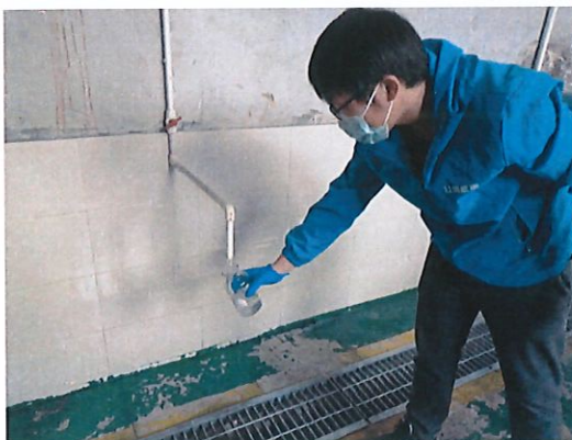
桃源加压站 (桃源镇) 采样口
